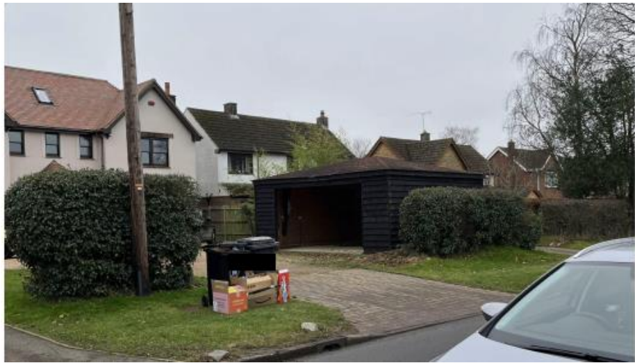
EXISTING SUMMER HOUSE
